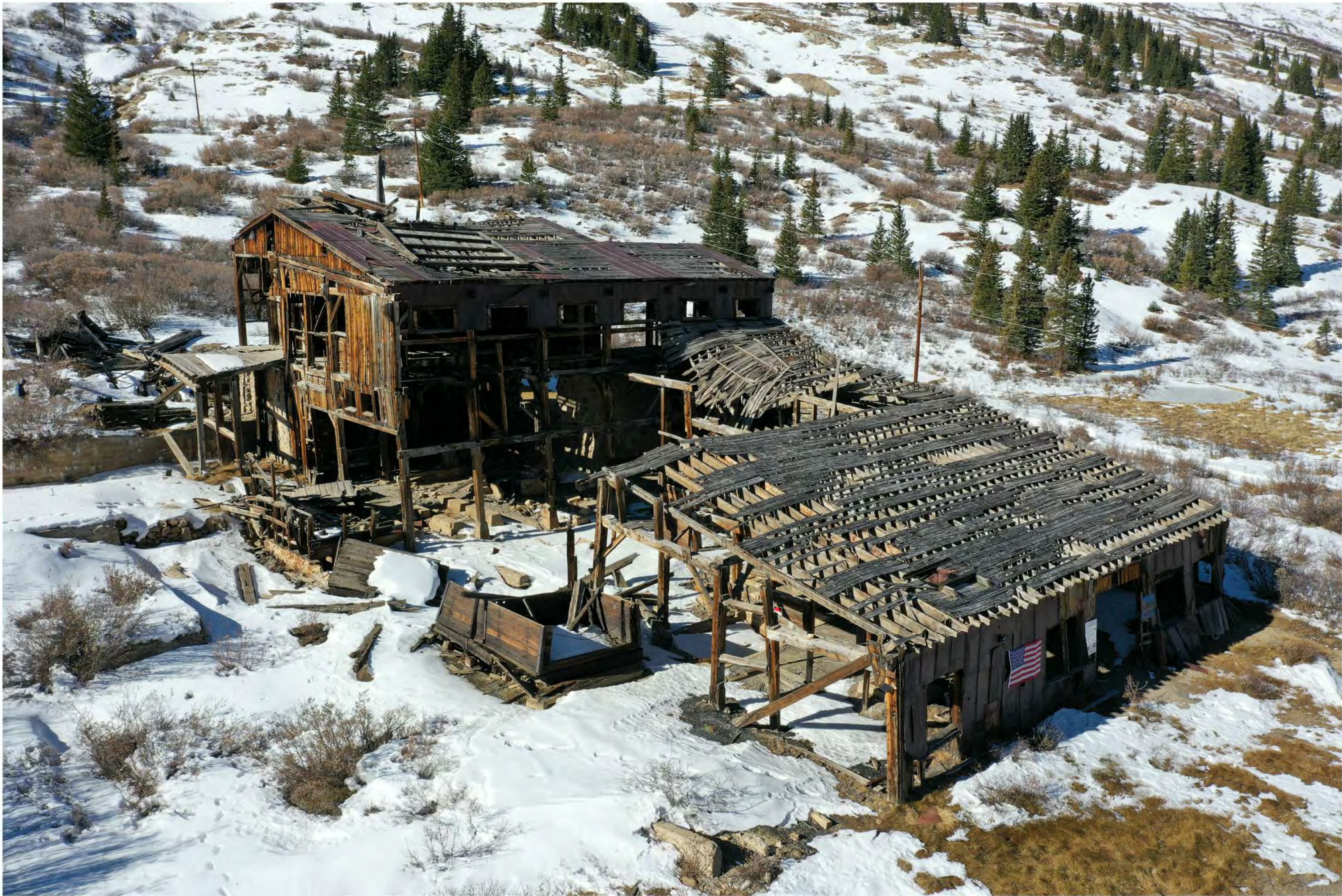
1 ROOF AERIAL S001 NO SCALE
